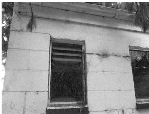
20. South Elevation – Horizontal cracks in masonry at lintel height
