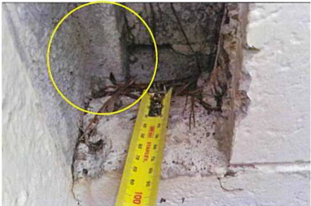
Figure 11 - Corbel detail (circled) observed as constructed on site
