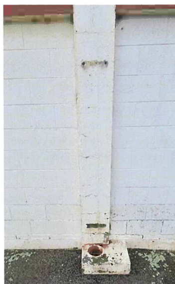
Figure 18 - Flexural cracking to concrete cantilevered posts
