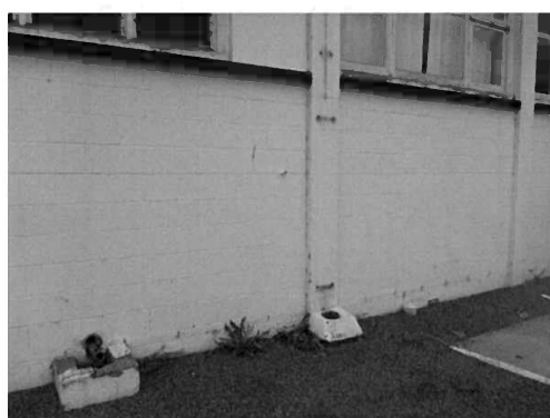
16. West Elevation – stepped cracks in masonry panels
