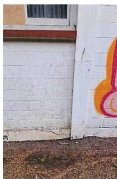
Figure 19 - Damage to foundation beam due to undermining of foundations unrelated to seismic damage
