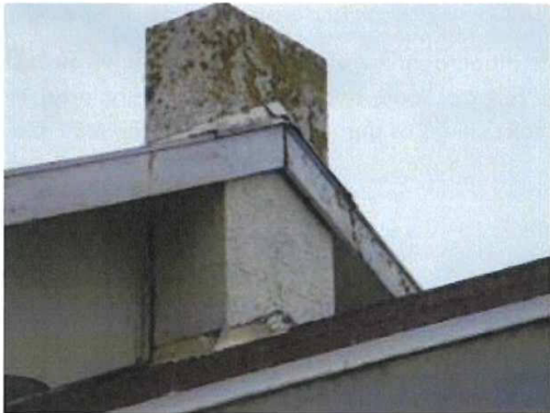
Figure 21 - Chimney damage from 2012 (Extracted from the Opus Report)
