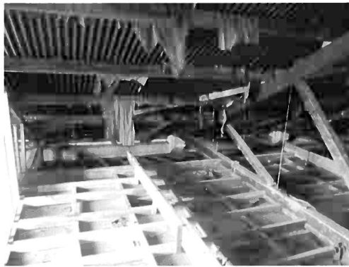
22. Truss supports and eaves beam
