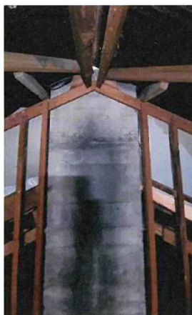
Figure 15 - As constructed chimney structure, tie back not observed.
