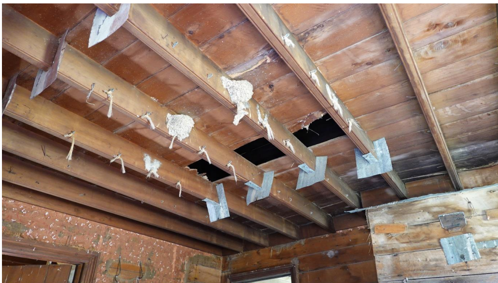
Figure 27. Nineteenth century cottage, detail of construction. Note hand-planed rafters.
