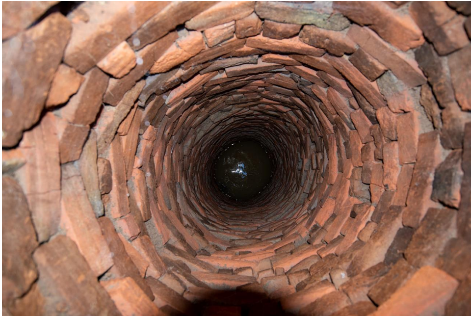
Figure 34. Brick-lined well interior. Top has concrete cover. Located southeast of mill site.
