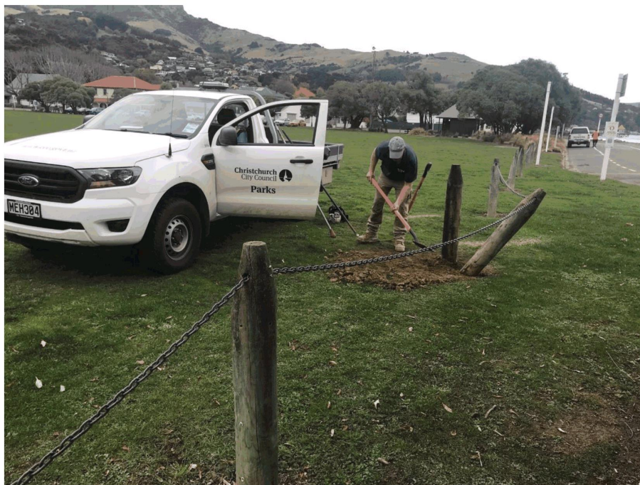
Akaroa Recreation Ground – replacing broken bollards.
