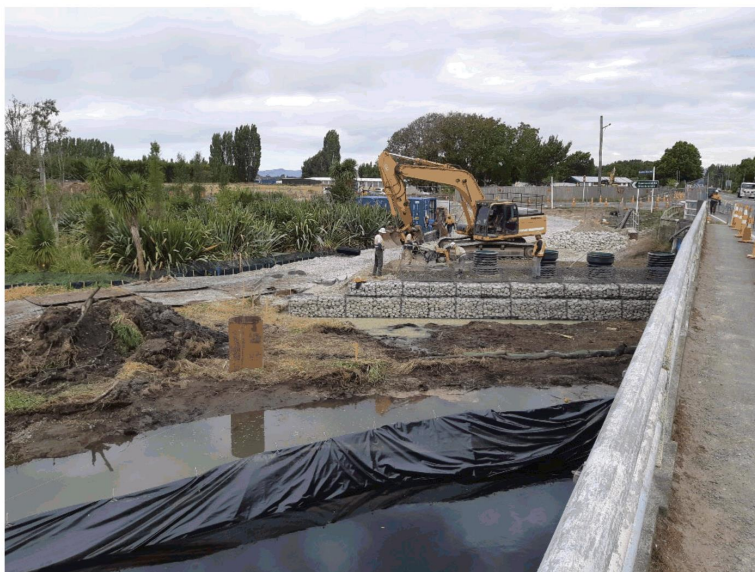
View from existing Bridge to South side of river Gabion Wall construction
