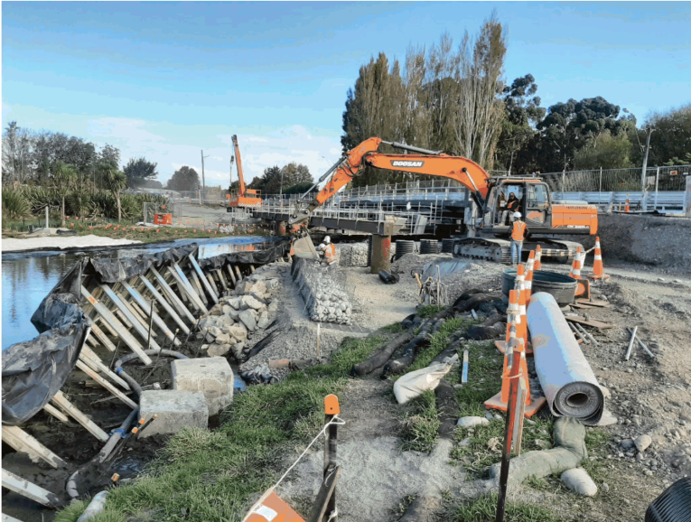
Gabion Wall construction North side of River
