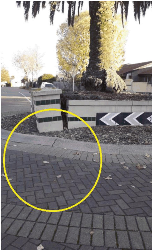
Photo 1) Tree 1 – Showing cracking and lifting in the pavement, possibly caused by the root system.
