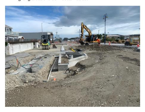
New V Channel, kerbing and one of the rain gardens on Eastern Side, preparation for Road carriageway
