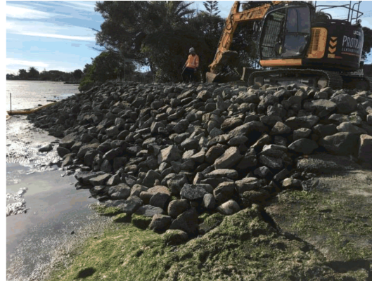
Rock wall strengthening at Heron Street (Southshore Emergency Bund Stabilisation Project)
