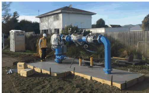
Inspection of the new above ground well head on Picton Well 3 by the well head security expert.
