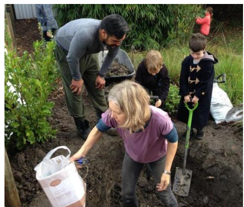
ENVIRONMENTAL: Volunteers building a household rain garden exemplar for treating stormwater
