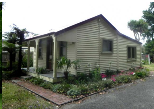
Kapuatohe Cottage 663 Main North Road, Belfast
