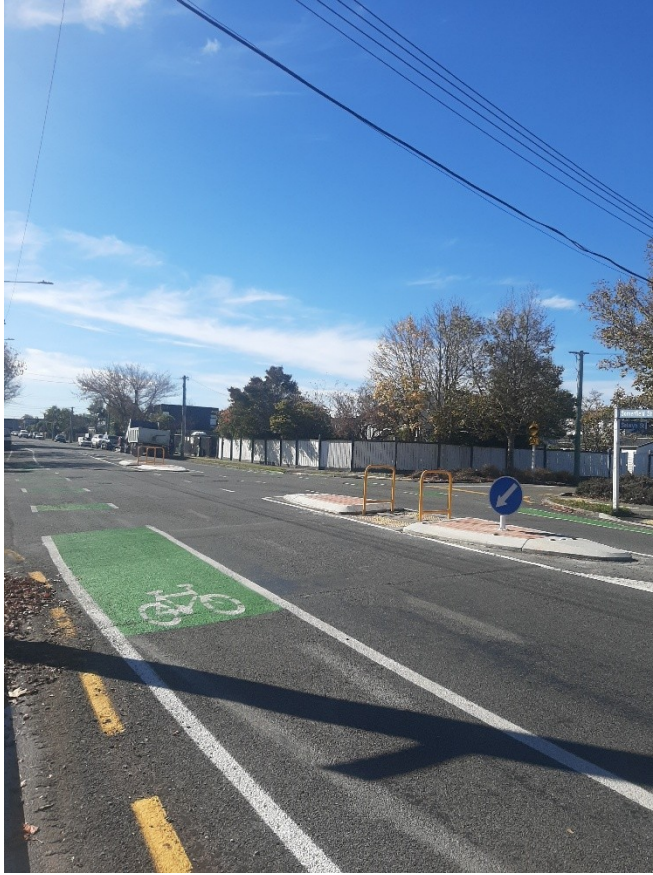
Above: Somerfield Street pedestrian safety
