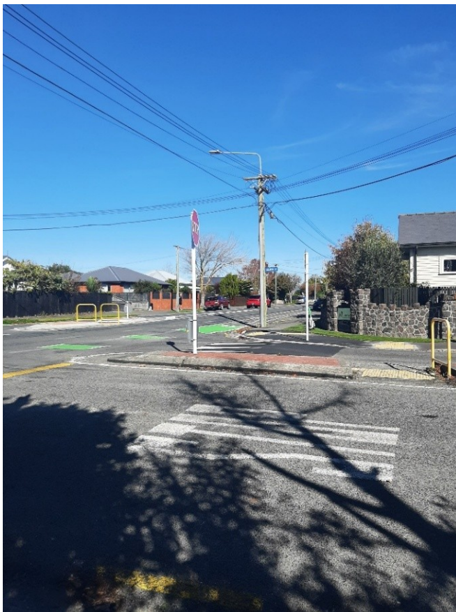
Above: Somerset Street and Selwyn Street intersection
