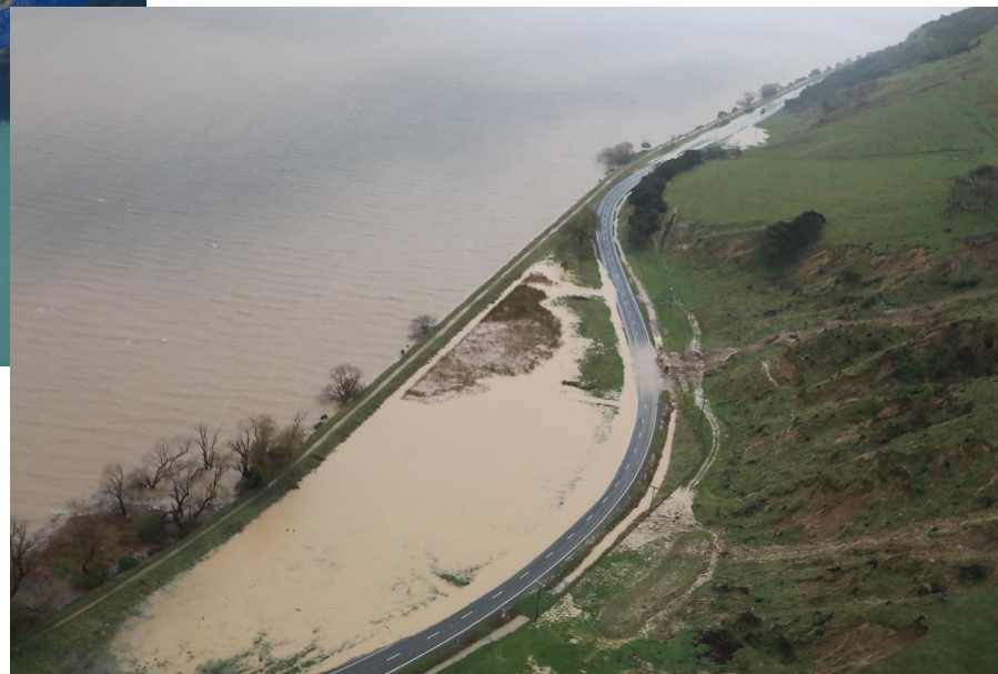
SH75 & Rail Trail near Little River
