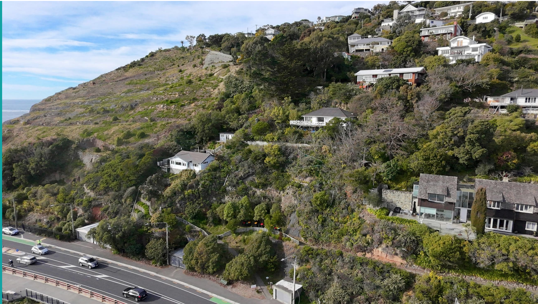
274a Main Road showing cliff at rear of site
