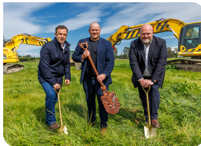
EcoGas staff Andrew Fisher, Andy Bedford and Jonathan West on site at the groundbreaking of the new Ōtautahi Christchurch Regional Organics Processing Facility.
