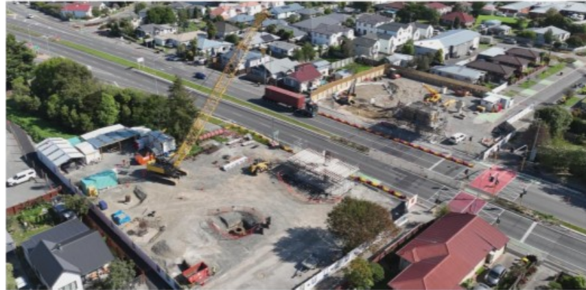
Construction of Brougham Street bridge.
