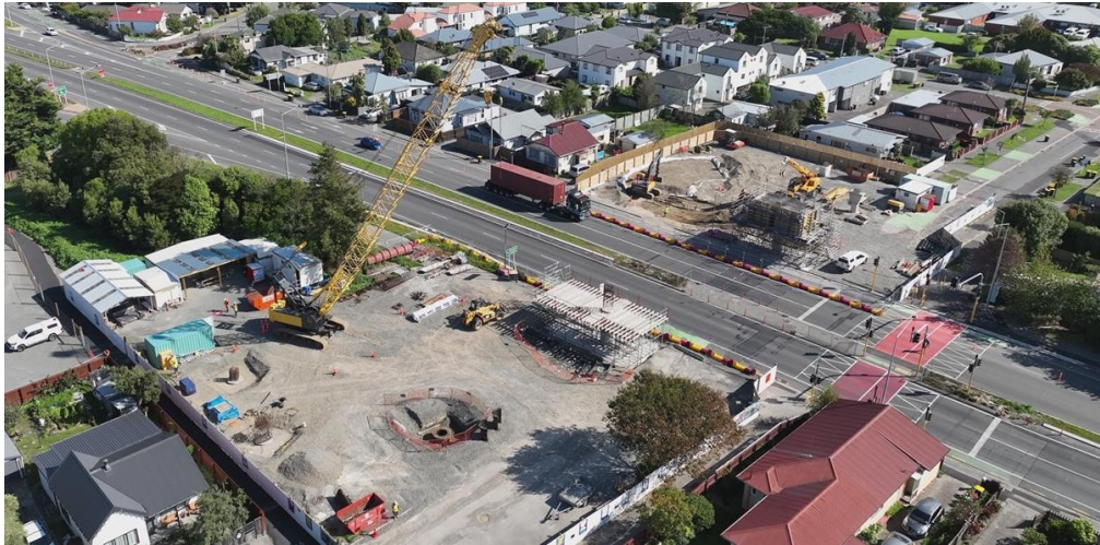
Construction of Brougham Street bridge.
