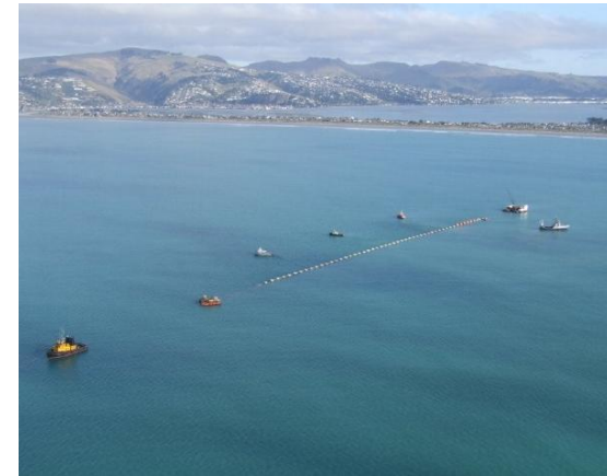
Installation of CCC outfall pipeline
