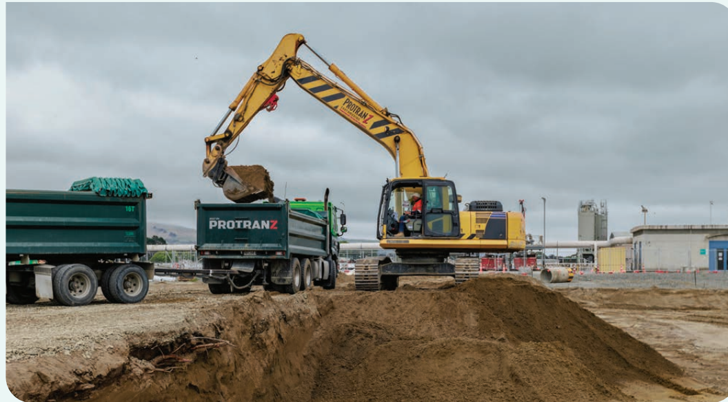
Activated sludge reactor construction charges ahead.
