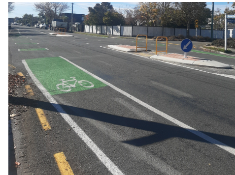
Somerfield Street Pedestrian Safety project
