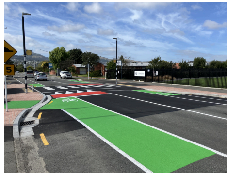
West Spreydon School Raised Crossing
