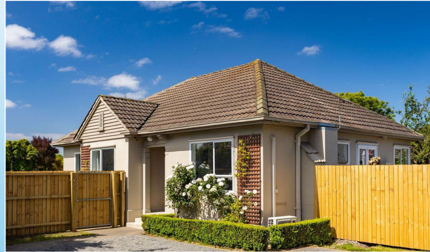
AIRMAN'S HOUSE NO. T4/3 37 SPRINGS ROAD
