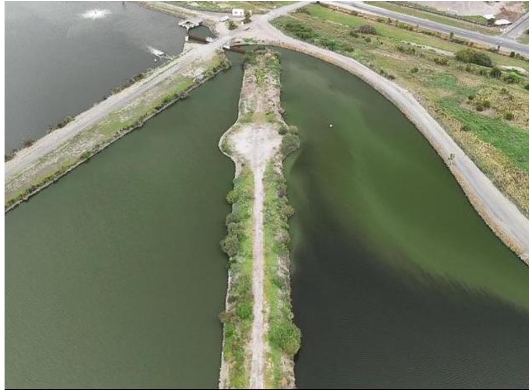
Wastewater Treatment Plant
