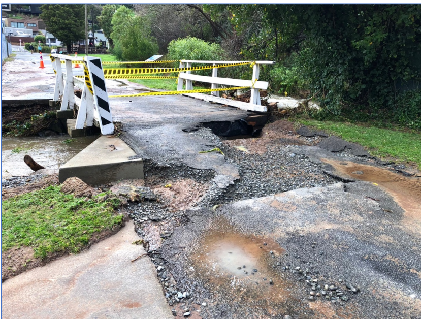
Bridge over Grehan Stream, Recreation Ground, July 27, 2022
