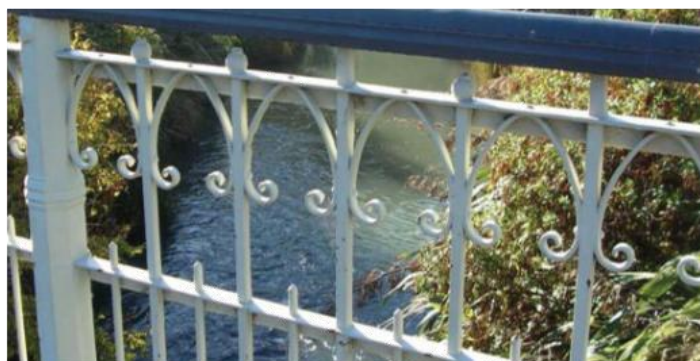
Historic bridge detail on Colombo Street bridge.
