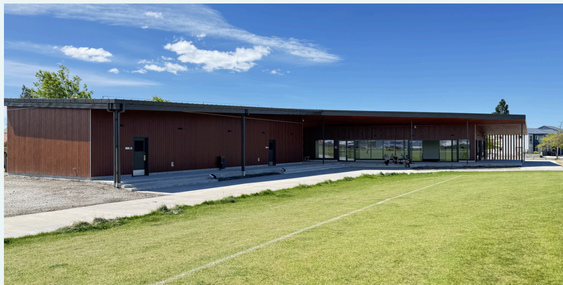
The new Lancaster Park Pavilion, which will open to the public in late November. The new facilities include changing rooms, a community centre with function and meeting spaces, and public toilets.
