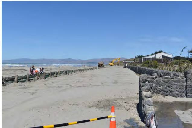
G. Existing stone retaining wall and existing sand fence to the left (under construction)
