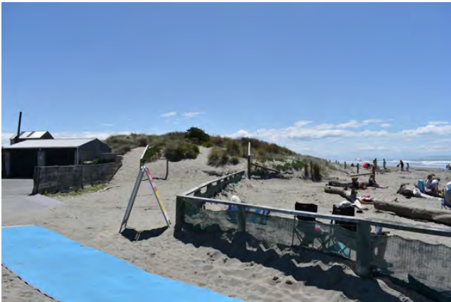
B. Existing sand dune timber retaining wall and wheelchair access matting leading towards beach
