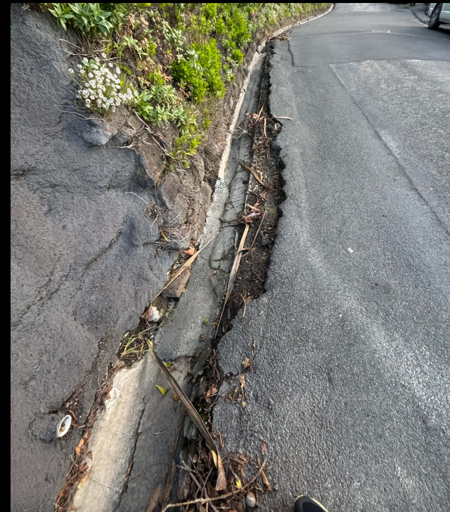
Photo uphill gutter - showing large areas of serious disrepair & wasted road space
