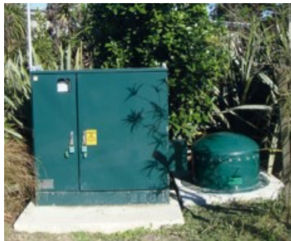
Electricity Cabinet and Odour Control Box
