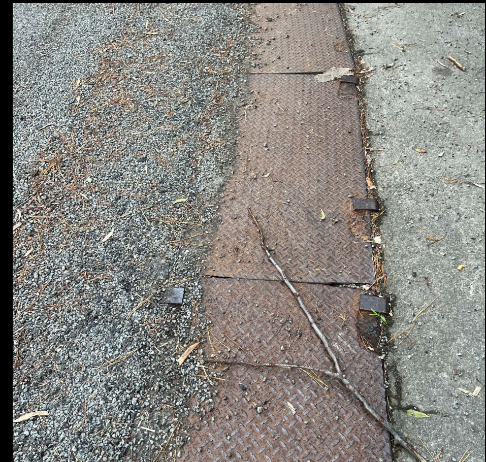
Example of gutter covers that were installed on various parts of Clifton Hill - To allow for improved & increased on road parking.
