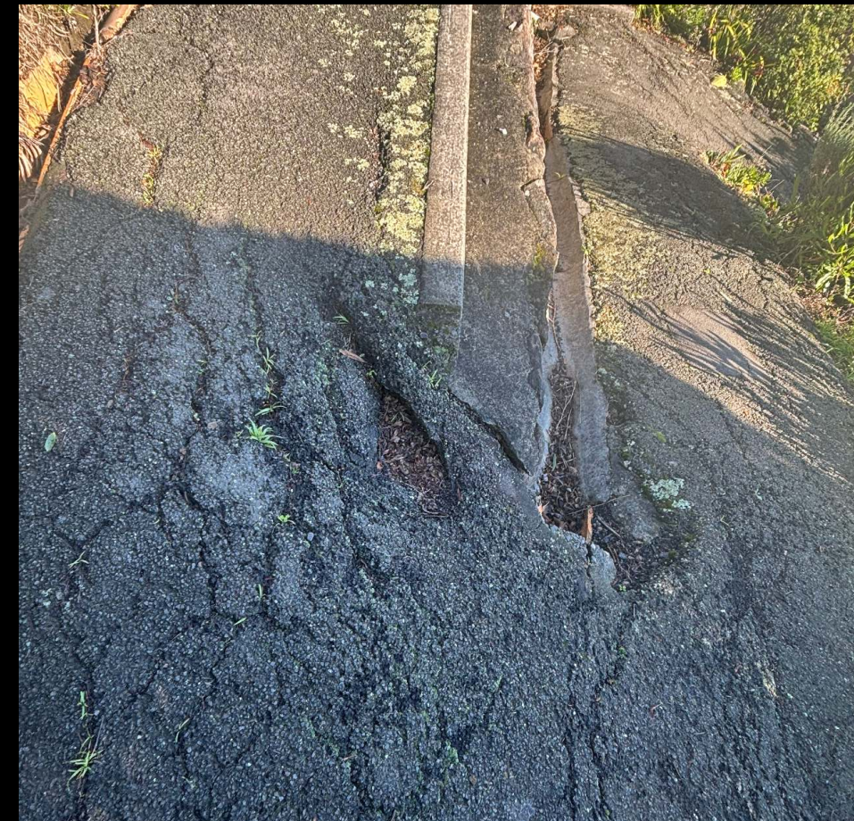
Walkway Photo - Showing uneven surface, cracks, no hand rails & general state of disrepair.
