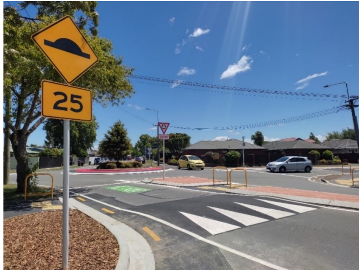
Speed hump treatment at Merrin/Withells intersection in Avonhead
