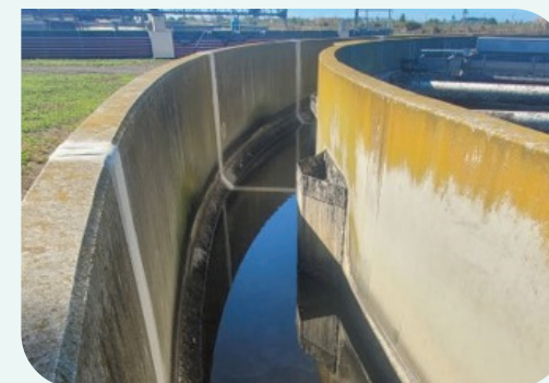
Clarifier - after repairs
