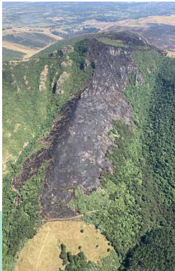
Ōhinetahi fire damage
