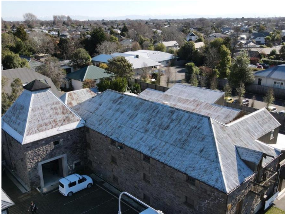
Aerial view of the Malthouse showing the extent of the roof requiring replacement (image provided by applicant)
