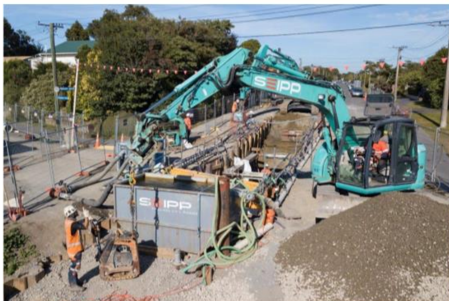
Pipe laying out of river crossing and down Malcom Ave
