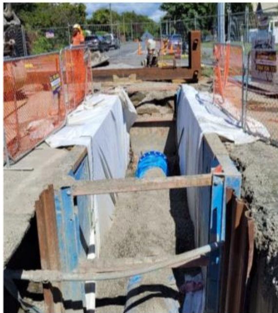
Crew coming to the end of Sandwich Road and sheet piling the corner
