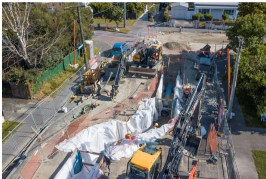
Crew on Birdwood Ave laying around the 45 degree dog leg
