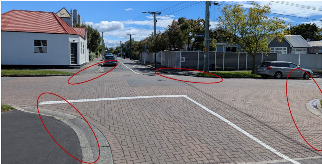
Image from scheme safety audit - Figure -1: Lack of yellow lines on the corners at the intersection of Perth St and London St (circled in red)
