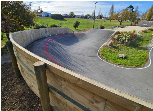
Above: Kyle Park, 1.2m solid panel fence.
