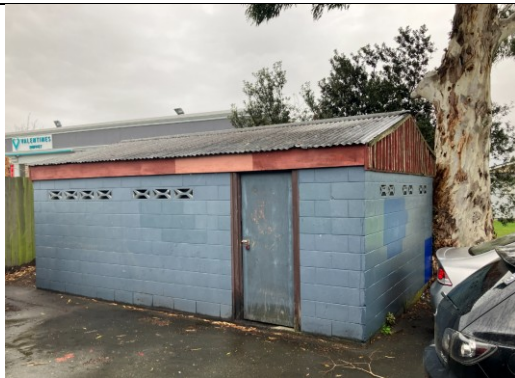
Figure 3: Photo of the shed.
