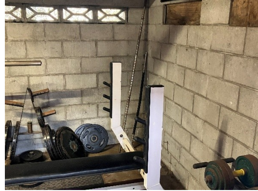
Figure 6: Image to show the overall brickwork from within the shed
