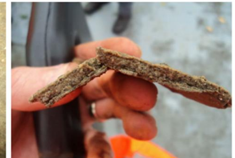
Figure 28 Sample of removed lining.
