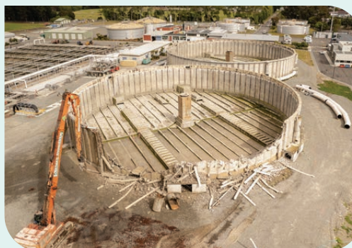
Demolition of the trickling filter tanks.
