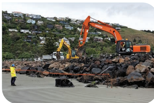
Sumner Esplanade rock revetment repair.
