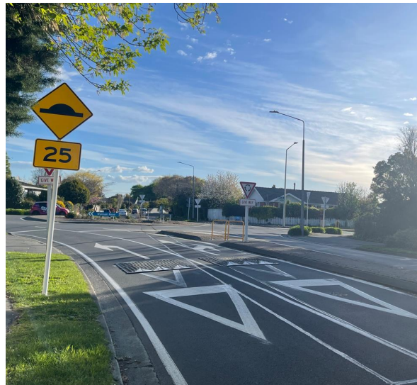
Figure 1: Photo showing installed speed cushions
