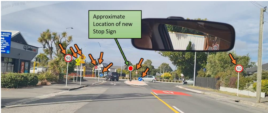
Figure 3-3: Signage visible to drivers on the McFaddens Road approach to the McFaddens Rd / Cranford St intersection
