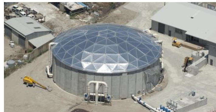
Aluminium cover replacing previous Glass Reinforced Plastic (GRP) cover
