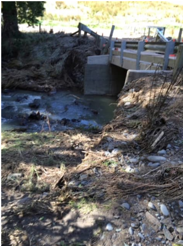
Holmes Bay Valley bridge upstream from the Holmes Bay bridge.
