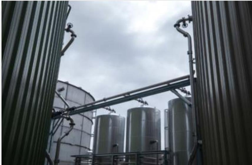
*Anaerobic digestion and storage tanks surrounding the pasteuriser: Reporoa OPF*
