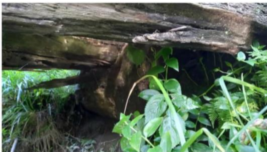
Figure 4 – decayed and splitting main beams near south abutment.
