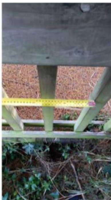
Figure 6 – 130mm spacing between balusters.
