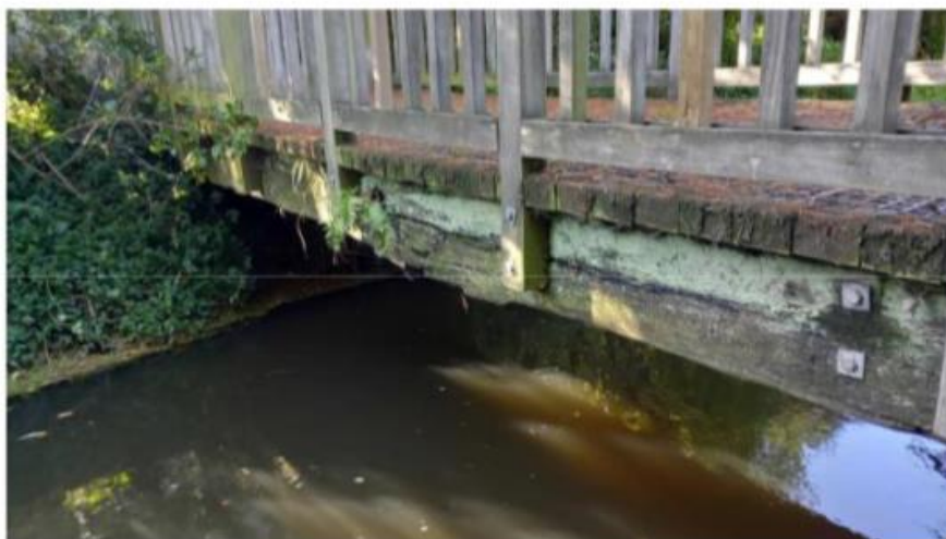
Figure 3 – decayed and broken beam on upstream side.
