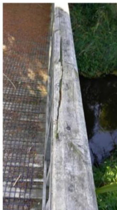
Figure 7 – splitting and rot beginning on handrails.
