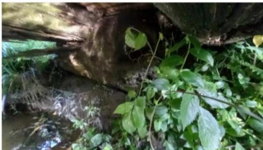
Figure 5 – shallow concrete abutment showing some undermining.
