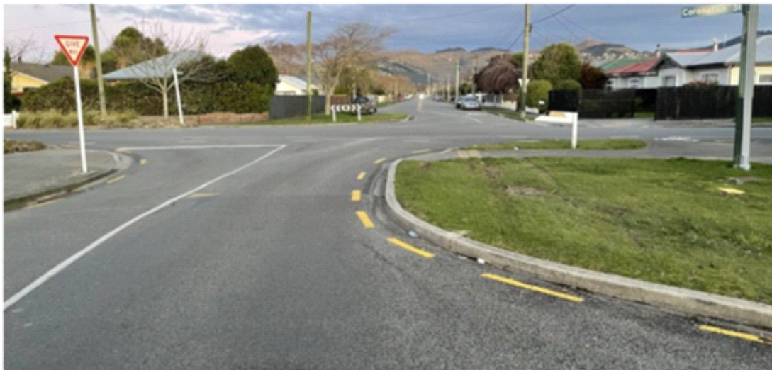
Figure 5: offset Coronation intersection and destroyed sight board - wheel tracks where high speed driver failed to slow
