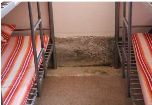
Figure 145: Exposed concrete walls and floor with evidence of some microbiological growth.
