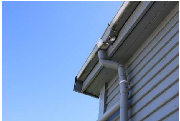
Figure 175: Failing guttering and downpipes.
