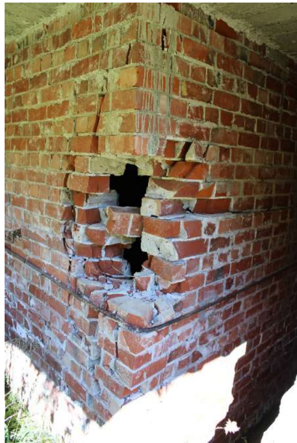
Figure 213: Damage to brick wall exterior.
