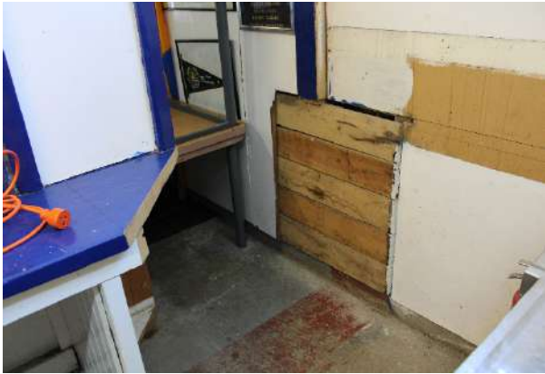
Figure 190: Covered hole in wall compromising weathertightness to building.
