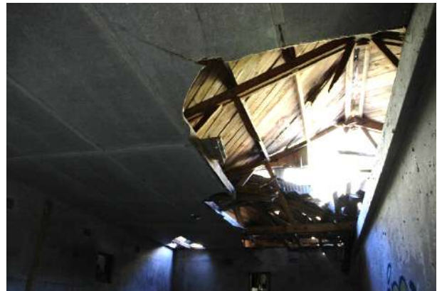
Figure 209: Roof penetration caused by rockslide.
