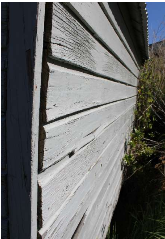
Figure 151: Condition of the store hut cladding
