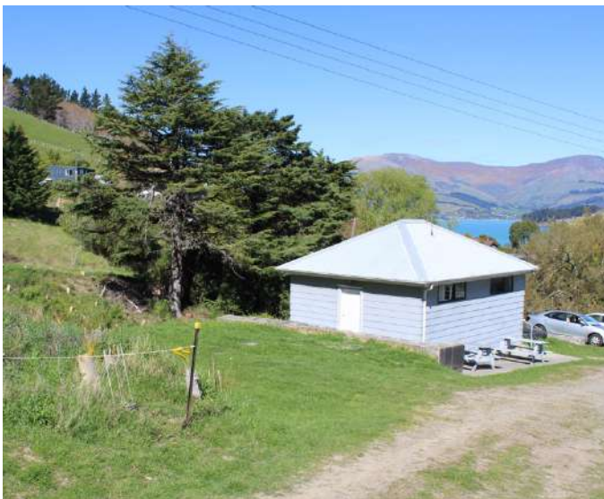
Figure 116: Car park area adjacent to the stream bank was filled some years ago without compaction and is now sinking.
