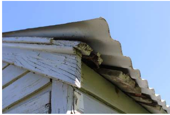
Figure 150: Condition of the store hut barge and fascia
