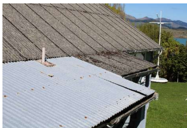
Figure 157: Severely deteriorated roof cladding.
