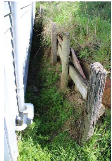
Figure 181: Failing retaining wall.
