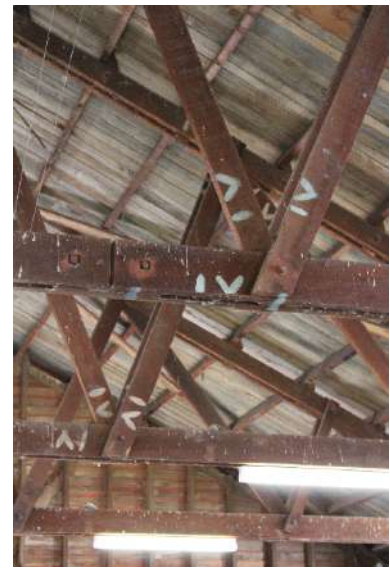
Figure 193: The 'numbered' pieces of the roof truss in the Drill Hall, taken apart and reassembled on site.
