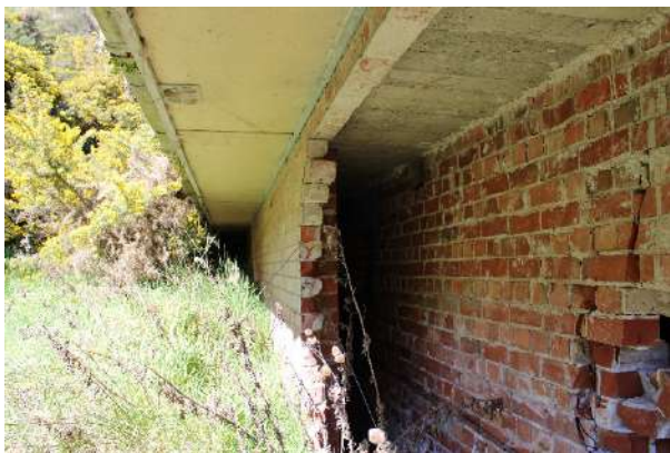
Figure 214: Damage to one of the magazine stores caused by a rockfall, exposing the separated double brick wall structure.
