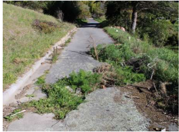
Figure 115: The subdivision road sealing is cracked, broken and overgrown with gorse, grass and weeds.
