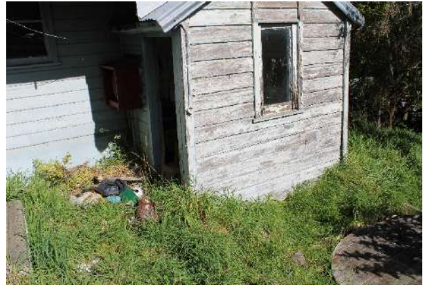
Figure 237: Gable end of the building showing flaking paint and rotten timber.
