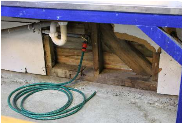
Figure 188: Exposed framing where internal linings have failed.
