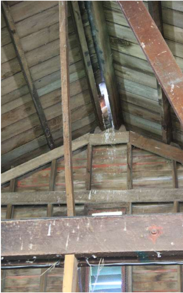
Figure 186: Evidence of pigeon infestation to roof and lack of weathertightness.
