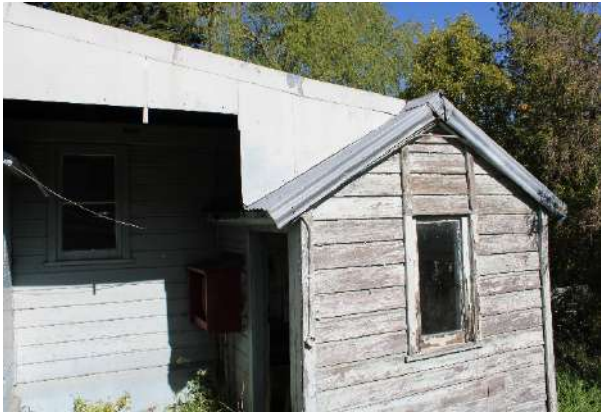
Figure 236: Gable end of the building showing flaking paint and rotten timber.
