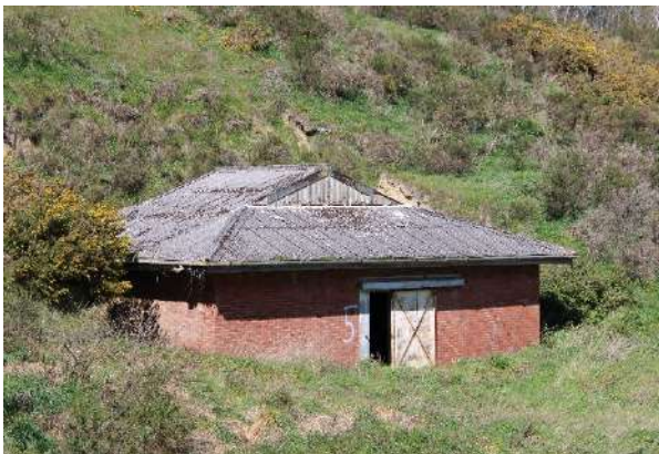
Figure 206: Severely deteriorated roof cladding
