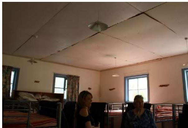
Figure 144: Suspended ceiling tiles failing.
