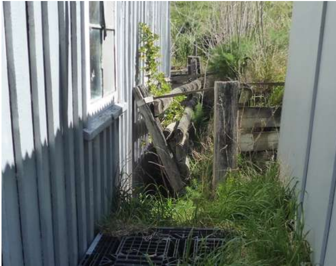
Figure 129: Timber retaining walls behind the Store, previously the Garage.
