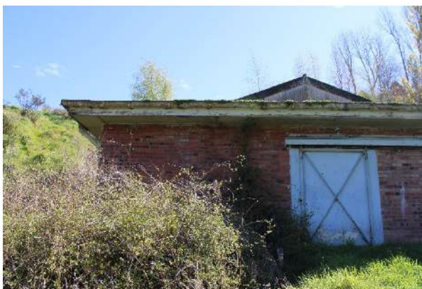
Figure 200: Microbiological growth to guttering.
