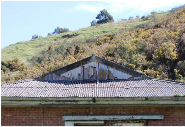
Figure 204: Severely deteriorated roof cladding
