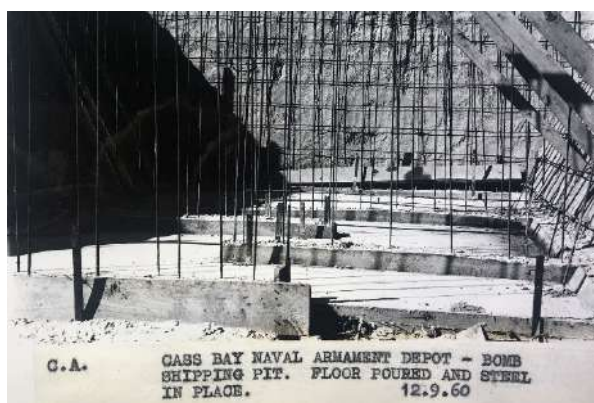
Figure 32: Cass Bay Naval Armament Depot – bomb stripping pit wall construction, 1960.
