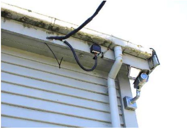
Figure 172: Microbiological growth to guttering.
