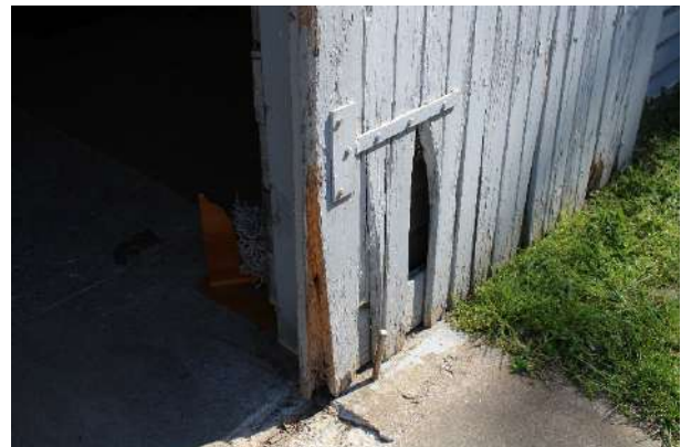
Figure 171: Damage to Drill Hall sliding doors.
