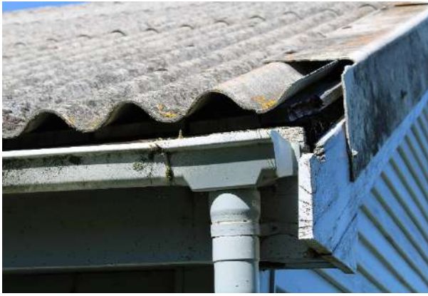
Figure 178: Severely deteriorated roof cladding.
