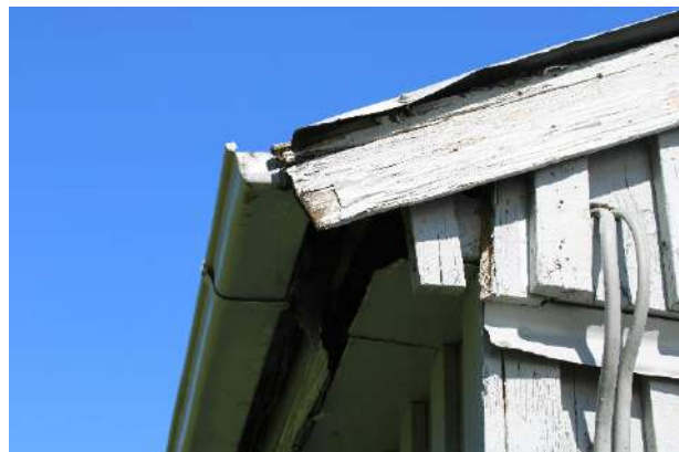
Figure 142: Rotten bargeboards and other roofing elements.
