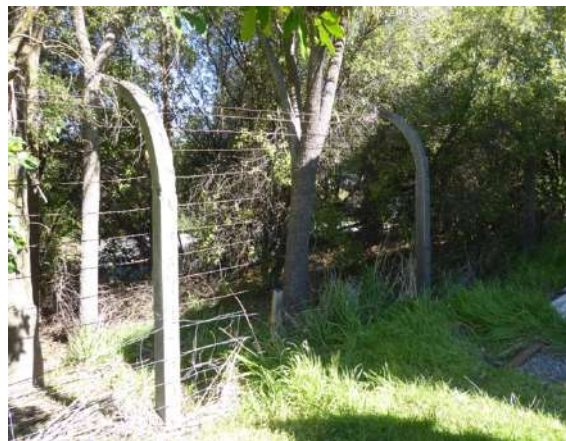
Figure 107: The 'unclimbable' curved concrete post and barbed wire boundary fence was installed to secure the naval armament depot and surrounds the entire site.
