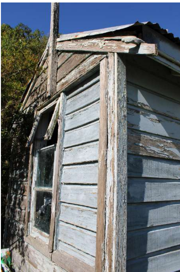
Figure 238: Rotten timber cladding and window framing to the exterior of the building.
