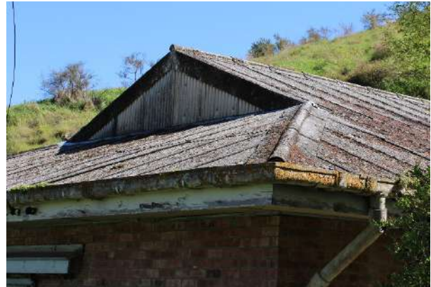
Figure 205: Severely deteriorated roof cladding and damage to guttering.
