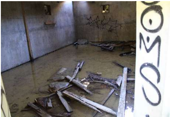
Figure 208: Flooding caused by roof penetration.
