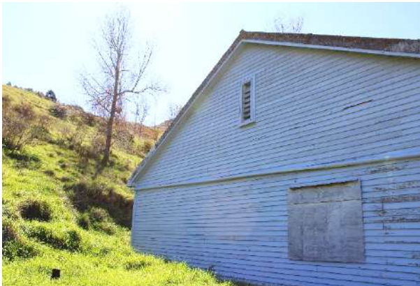
Figure 176: Severely damaged bargeboards, flaking paint exposing timber beneath, plywood covering hole in the building.
