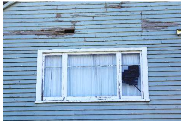
Figure 162: Missing timber allowing moisture to enter the building and broken window.
