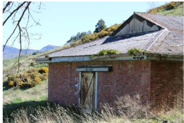
Figure 207: Biological growth to guttering.
