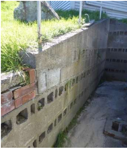
Figure 131: Concrete block and brick retaining wall behind the Ward Room requires inspection..
