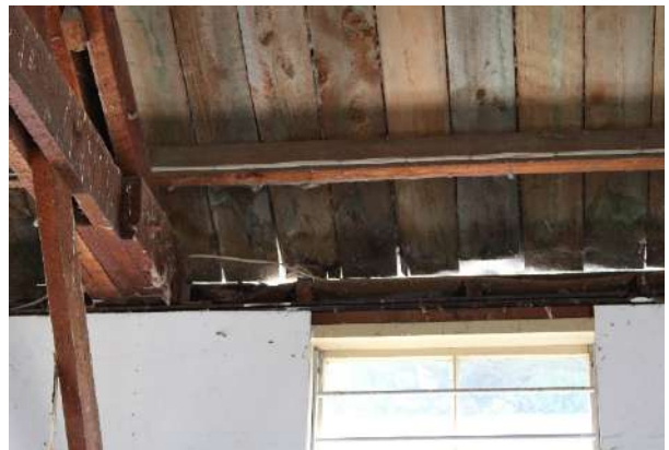
Figure 183: Lack of weathertightness to roof edges.
