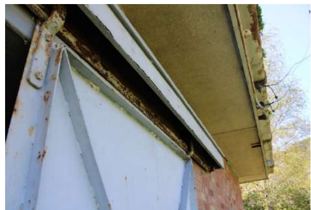
Figure 201: Corrosion to steel sliding doors.
