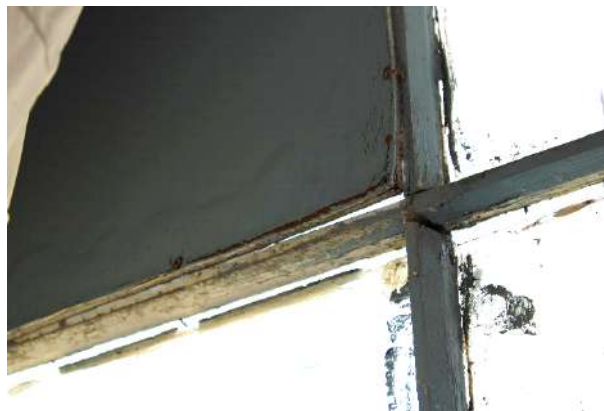
Figure 146: Window glazing bars failing and boarded over in some areas.
