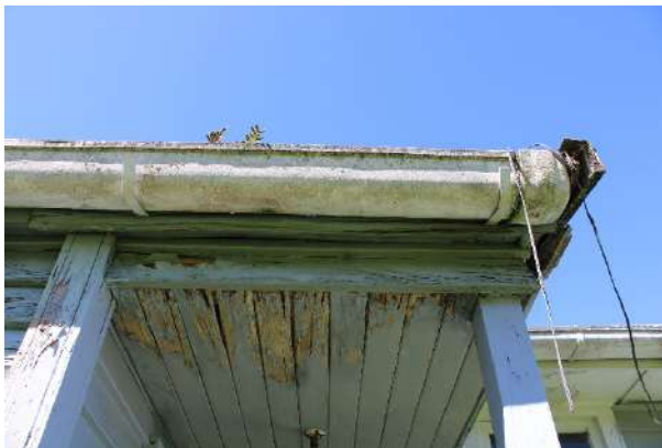
Figure 161: Rotten timber and failing guttering.
