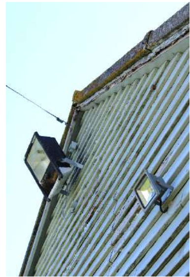
Figure 160: Paint flaking exposing timber underneath to elements.
