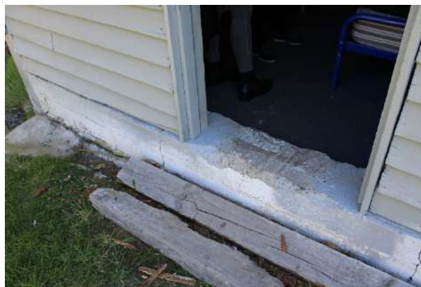
Figure 148: Entranceway with timber planks in the place of stairs.
