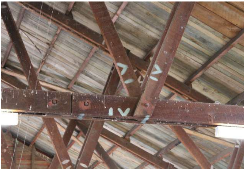
Figure 192: The 'numbered' pieces of the roof truss in the Drill Hall, taken apart and reassembled on site.
