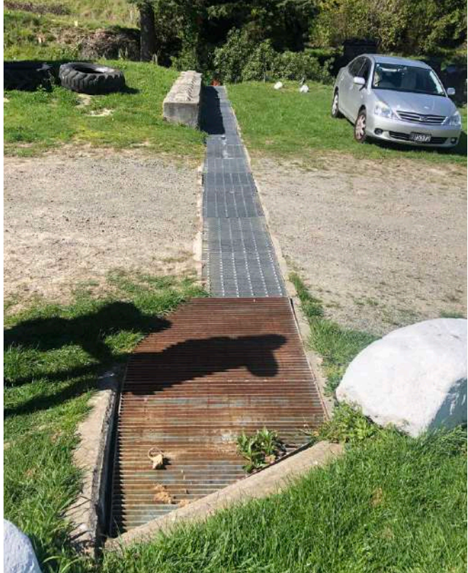
Figure 95: Drainage issues are evident with historic and recent drainage channels constructed on the site.
