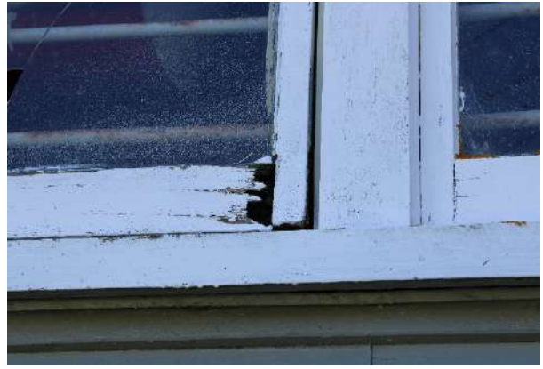
Figure 173: Damage to timber window frames.
