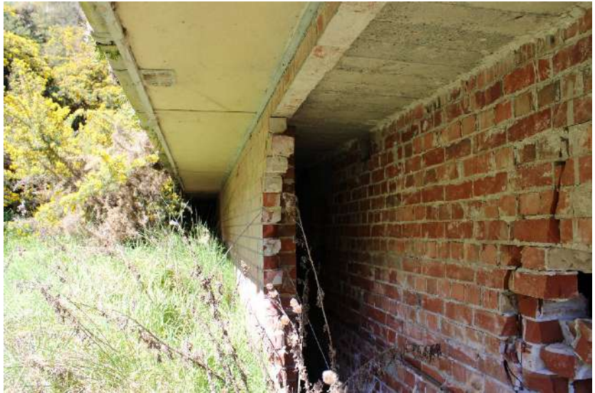
Figure 211: External damage to double layer brick wall caused by rockslide.
