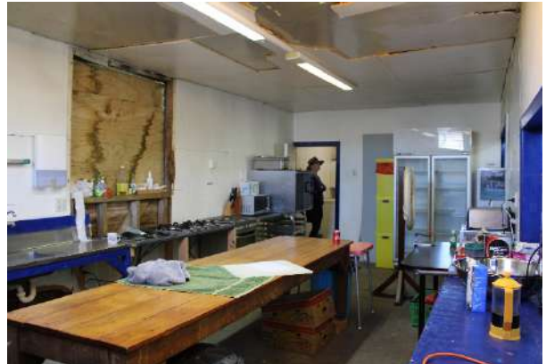
Figure 189: Kitchen with exposed concrete floor, failing ceiling linings, and external hole covered with plywood.
