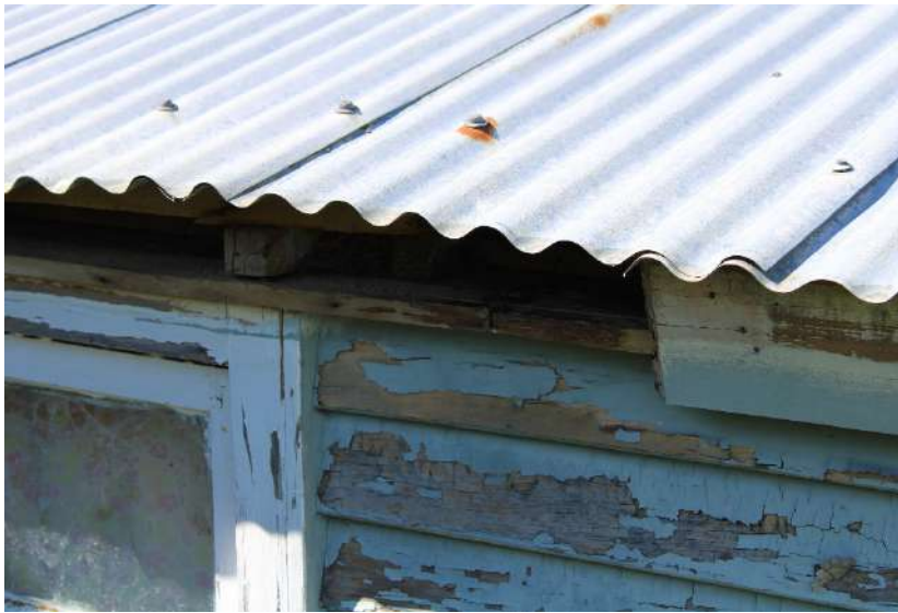
Figure 159: Paint flaking exposing timber underneath to elements.
