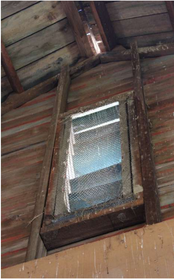
Figure 184: Evidence of pigeon infestation to gable end external grilles.
