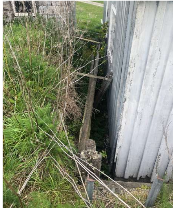
Figure 136: Retaining wall between the Garage and Small Store is falling apart.
