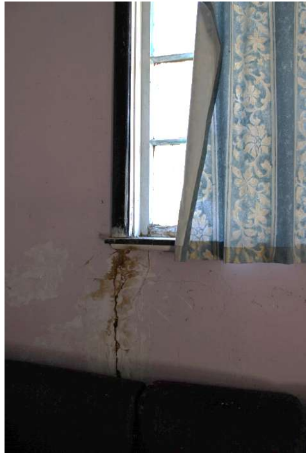
Figure 229: Severe wall cracking and window damage.
