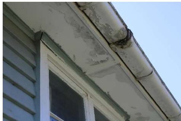
Figure 164: Failing guttering and subsequent water damage to soffit.
