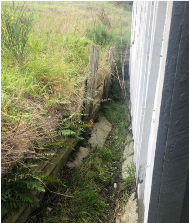
Figure 135: Behind the Garage - deteriorating retaining wall.
