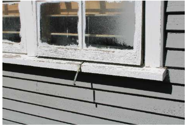
Figure 179: Damaged timber window frames.
