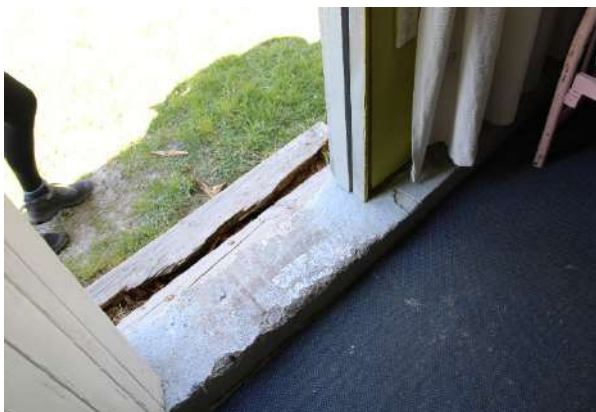
Figure 147: Entranceway with timber planks in the place of stairs.
