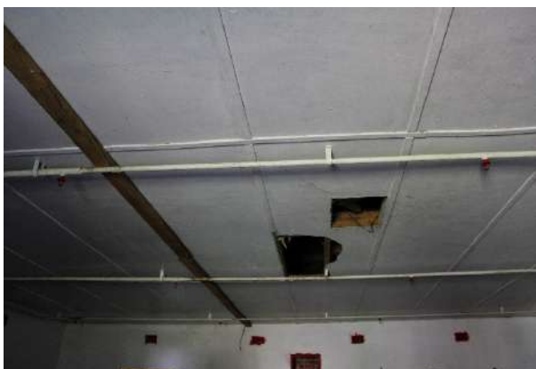
Figure 202: Failing internal linings.
