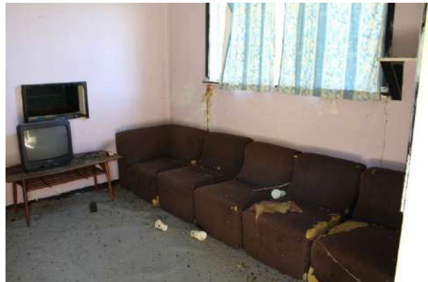
Figure 227: Interior of laboratory building showing severe pigeon infestation and failing wall/floor/ceiling linings.
