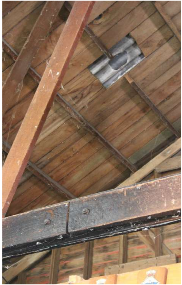
Figure 187: Charred beam from historic fire, and covered hole in the ceiling where chimney originally existed.
