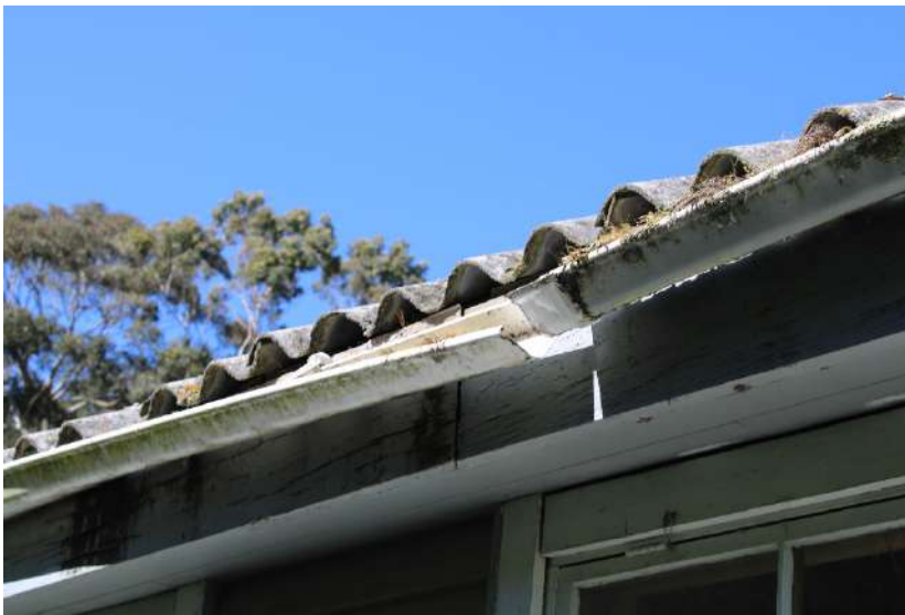
Figure 180: Failing guttering.
