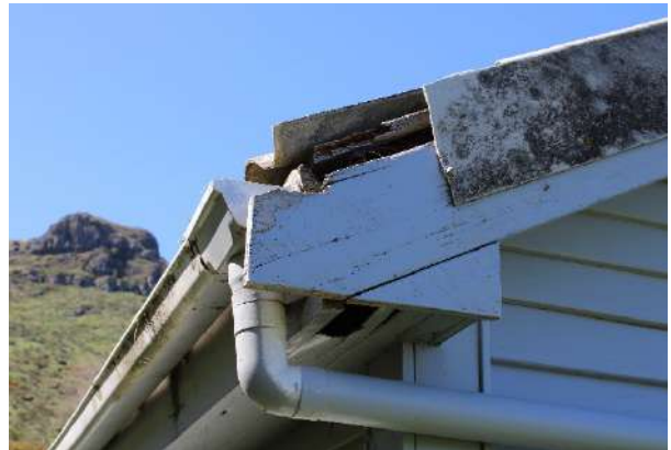
Figure 177: Damaged bargeboards and roof cladding, rotten timber below.
