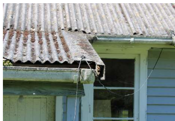
Figure 158: Severely deteriorated roof cladding.
