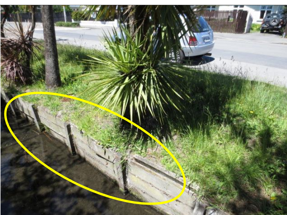
Figure 2: Cabbage Trees and damage to drain, 9 Aylesford Street.
