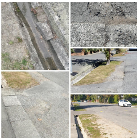
Konini St potholes, crumbling kerbs, & berm erosion.
