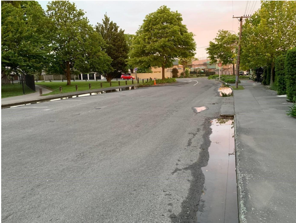
Photo 2: Titoki street flooding after rain. In addition, there is severe ponding when it rains, even though the sumps have recently been cleaned out. The entire street would benefit from new stormwater infrastructure, new kerb and channel and a wider footpath on the northern side to cope with heavy pedestrian counts weekdays from school students and weekends for the Farmers market. There is also an option to add a cycleway/ footpath link from the University cycle lane at Riccarton Bush to Westfield mall.
