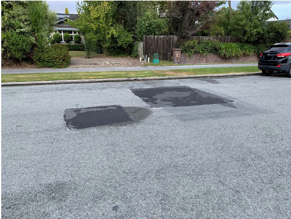
Photo 3: Subsidence outside 23 Rata street. For several years now the subsidence on Rata street has been filled with hot mix rather than investigating and remedying the below surface cause. Most likely this is a failed sewer lateral repair carried out previously.
