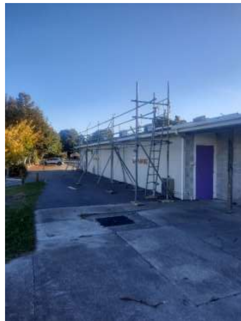
Scaffolding and edge protection in place
