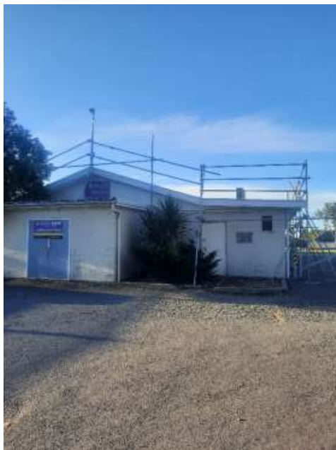
Scaffolding and edge protection in place
