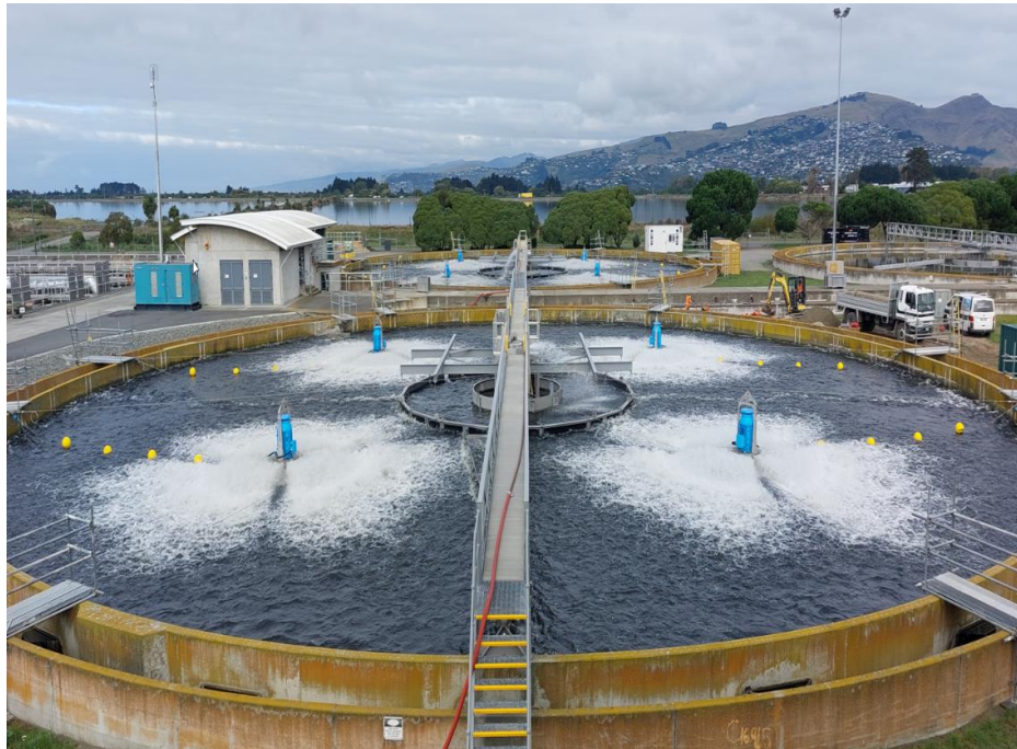
Aerators on the existing clarifier tanks which have been converted into aeration basins for wastewater treatment
