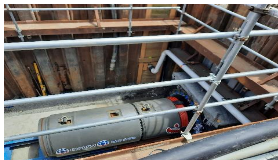
Pipe jacking under the railway lines is in progress
