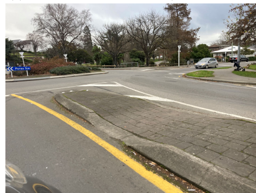
Barrington / Cashmere: Grey concrete and pavers
