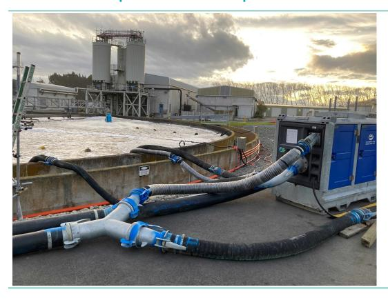
The temporary pumps that were set up to pump-over from the aeration basins (converted clarifiers) to the existing clarifiers to support early growth of the sludge biomass are being disestablished as the 16 new permanent pumps are installed (commissioning in July).
