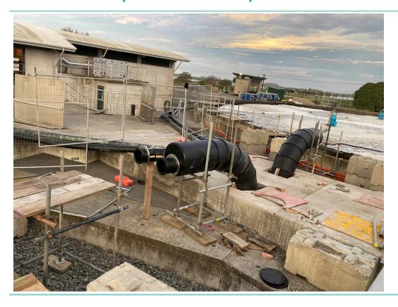
The new pipework between the aeration basins (converted clarifiers) and the channels leading to the existing clarifiers is being installed.
