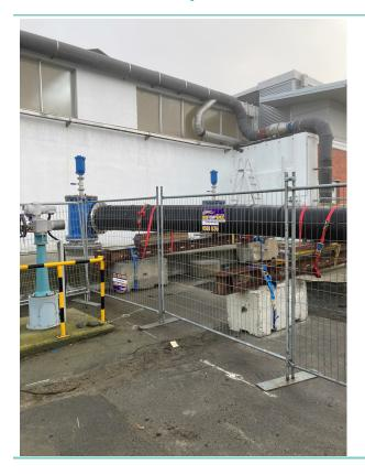
Work complete on the trickling filter by-pass pipe and testing underway.
