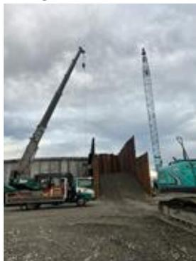
The Insurance Subcommittee visited the Wastewater Treatment Plant again to see the progress towards removing the biomass from the trickling filters (ramp being built on left) and the installation of temporary pumps that are providing the much-needed aeration in the tanks before the wastewater enters the oxidation ponds (right).
